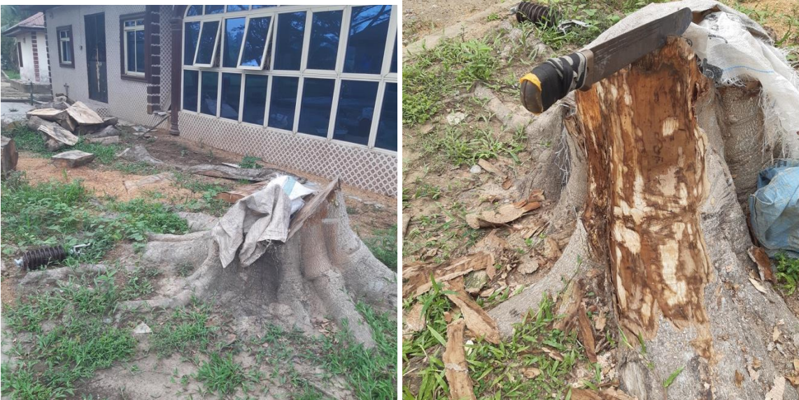
Figure 3: This tree with buttress root have been cut down because of the damages being caused to the foundation of the nearby building
