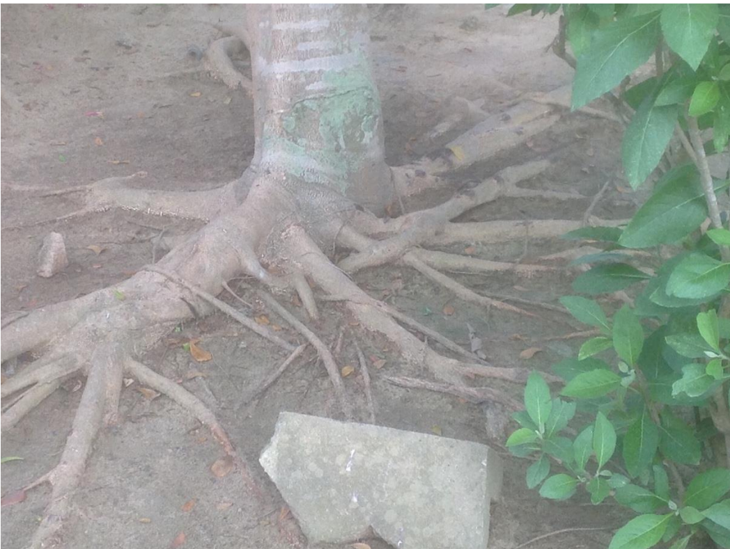
Figure 2: Buttress root system causes huge damages to infrastructures
